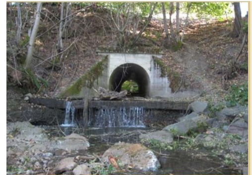
Jones Creek railroad culvert before improvement.
