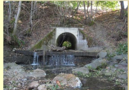
Jones Creek railroad culvert before improvement
