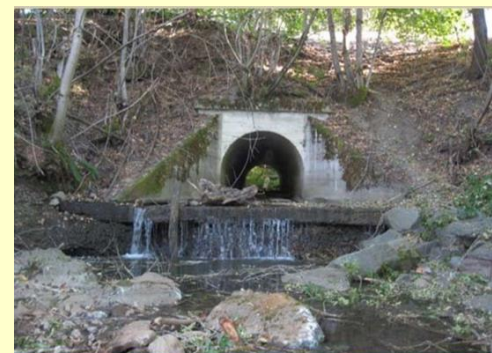
Jones Creek railroad culvert before improvement.
