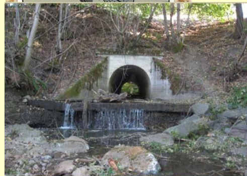
Jones Creek railroad culvert before improvement.
