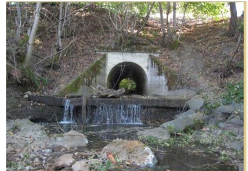
Jones Creek railroad culvert before improvement
